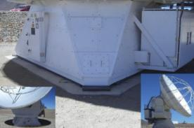
Figure A.2: Structure of an antenna pad (actual pad at the OSF) (left) and detail of antenna anchored to a pad (right).
