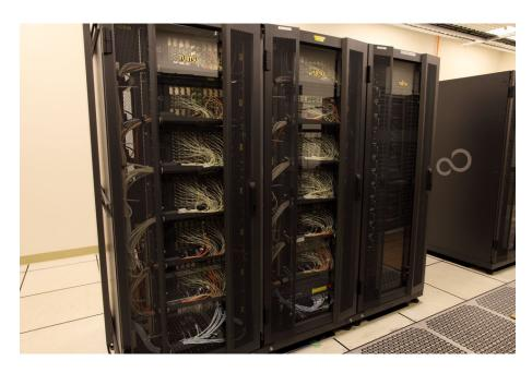
Figure 5.4: Two quadrants of the ALMA Compact Array (ACA) correlator installed in the ACA correlator room. Credit: ALMA (ESO/NAOJ/NRAO), S. Okumura
