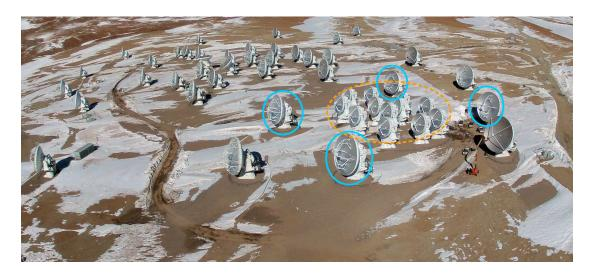
Figure 2.1: The ALMA 12-m Array in its compact configuration (left hand side of the image). The ACA with all 7-m antennas (dashed orange circles) and four single-dish 12-m antennas (blue circles) are distributed in the right hand side of the image. A few unoccupied stations can be seen, to which antennas of the 12-m Array can be moved by the transporter as the array is being reconfigured. At its most extended configuration, antennas in the 12-m Array will be about 16 km apart.
